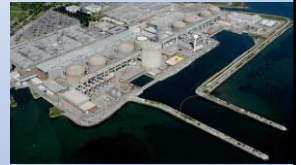
There are currently 18 commercial nuclear power plants in Canada. Pictured here is the Pickering generating plant in Pickering, Ont.
